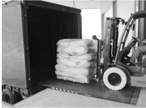
Dock leveller in operation
